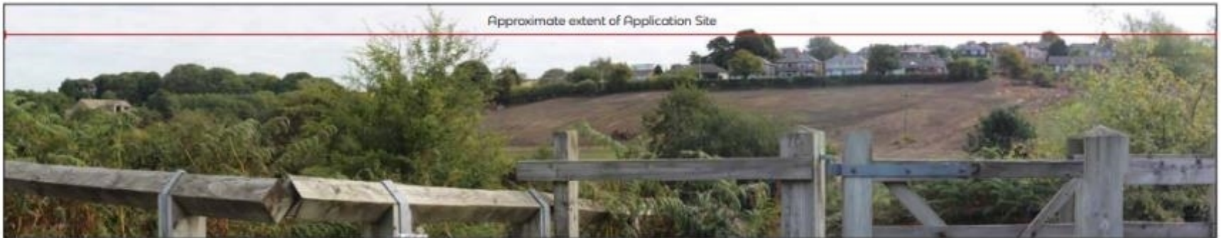
Photoviewpoint 1: Taken from Blackburn Brow and the entrance of the Chorley Loop towards the direction of the site Distance from site: 80m Coordinates: X: 359112 Y: 419709
